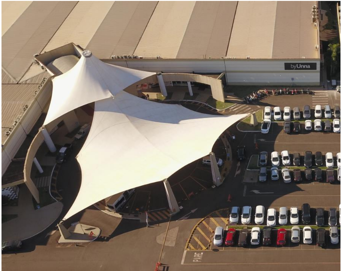
Obra: Shopping Avenida Fashion- Maringá- PR
